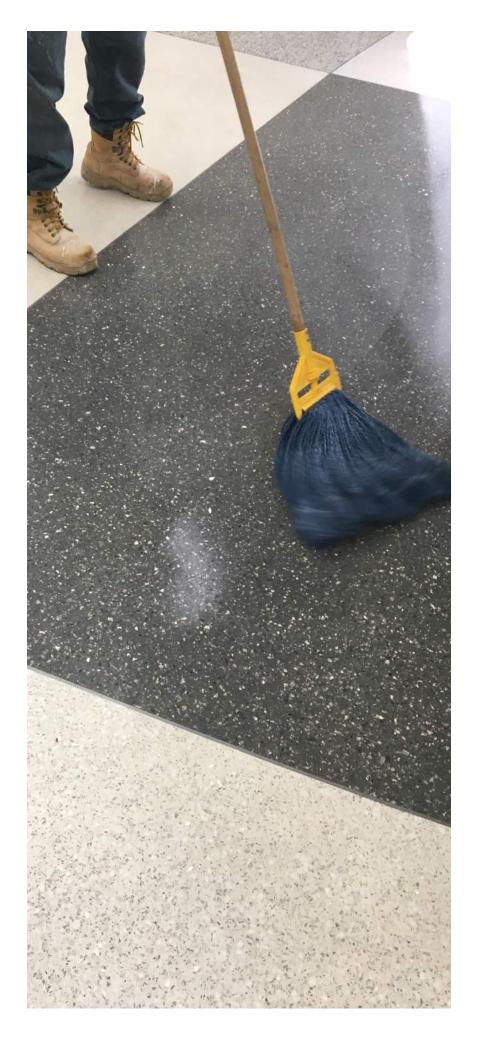
An epoxy terrazzo floor is easily maintained due to its hard surface and absence of grout joints and seams.
